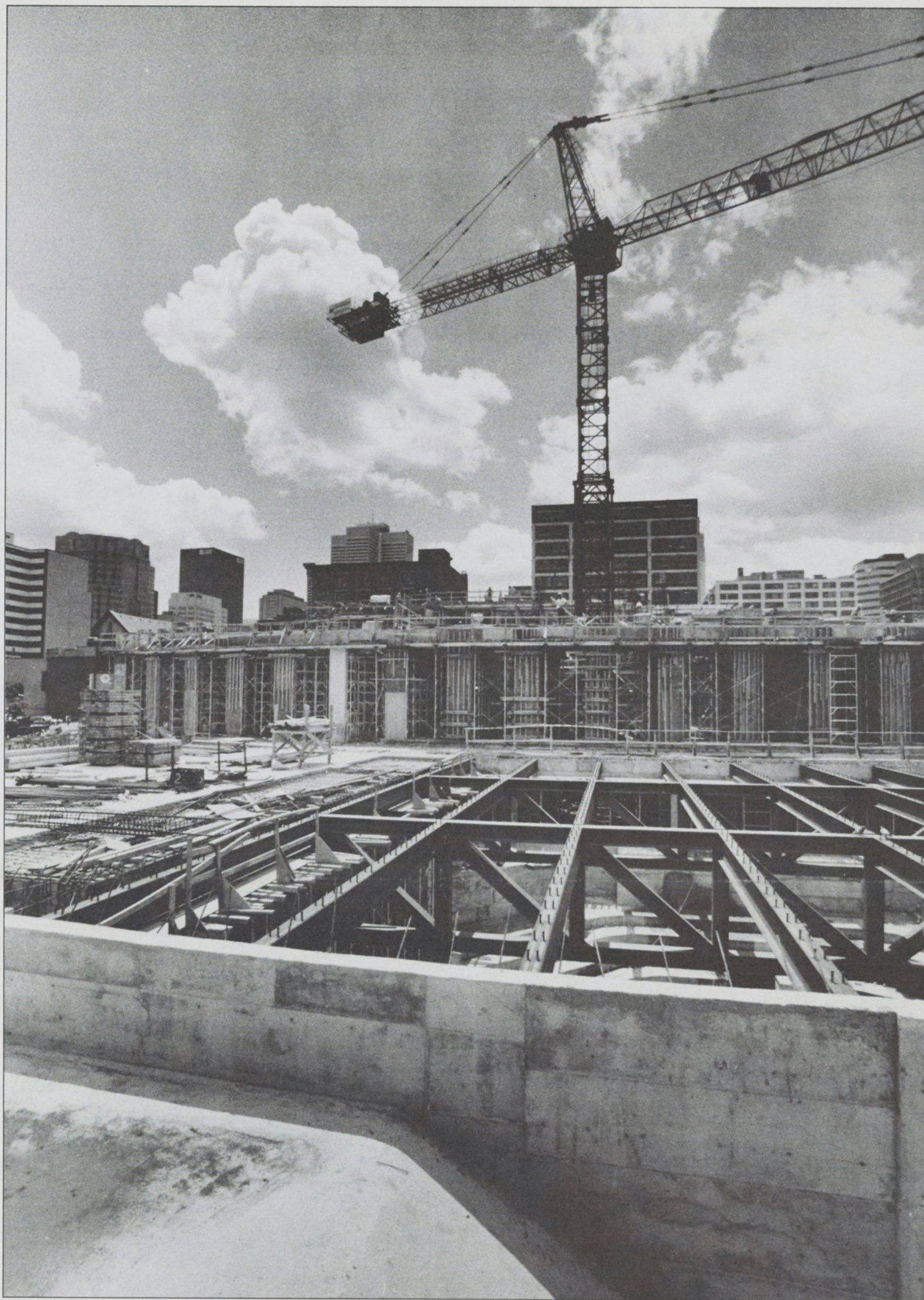
Construction site, July 10, 1990. Photo: Denis Farley.
