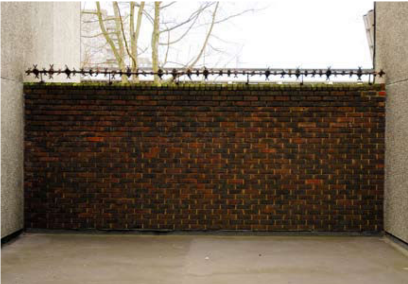
Wall with Razor Wire, Thamesmead South, London, 2006
